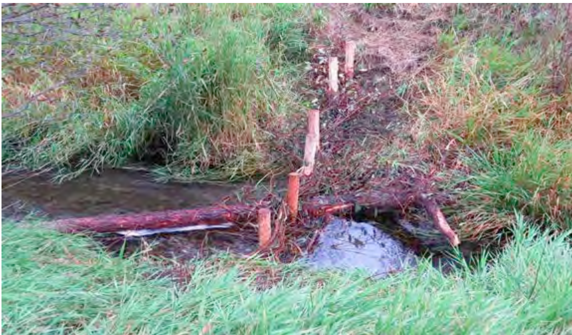
Figure 78: BDA – Two pilings extending onto the bank with LWD placed through the structure
