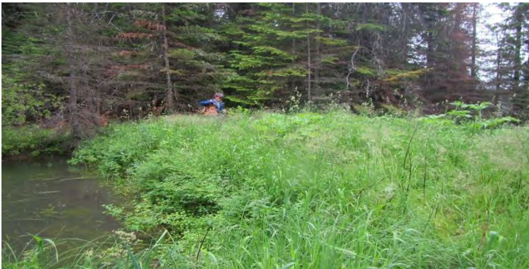
Figure 57. Earthen BDA and Wetland Cell in second growing season after construction.
