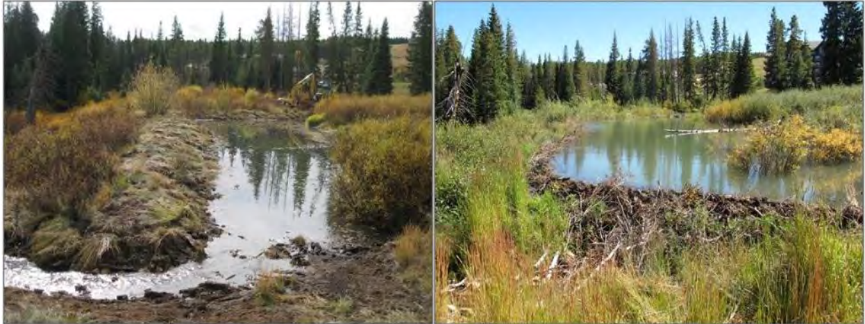
Figure 73: The left photo shows a repaired beaver dam and pond just after construction in 2012 with a single "spillway." Beaver dammed the spillway in 2013 and continued to raise the height of the dam in 2014 (right photo).
