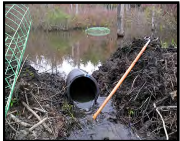
Figure 40: Flexible pond levelers with cylindrical wire cages on the upstream pipe end. Clockwise from upper left (a) and (b) are examples during the construction phase, while (c) is an example just after completion but before dam repair. (b) is a downstream view of a pond leveler after beaver have repaired the dam. Photographs from Boyle (2006).
