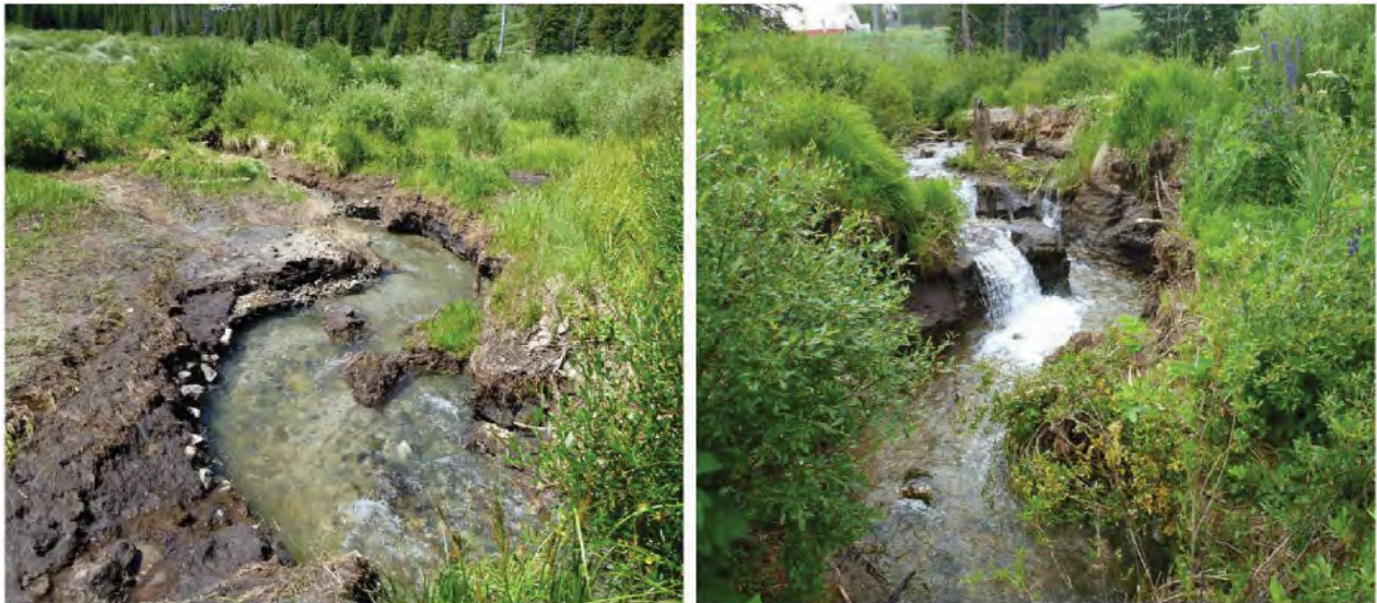
Figure 62: Once dams failed, a channel formed and immediately began head cutting. These photos show the Boreas Creek channel in different stages of incision, initial channel formation (left) and advanced incision (right)
