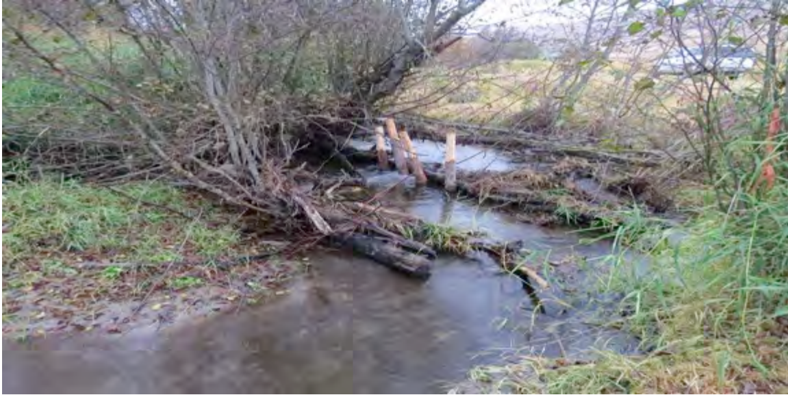
Figure 79: Partially channel spanning BDAs and LWD additions to a naturally occurring log and debris jam
