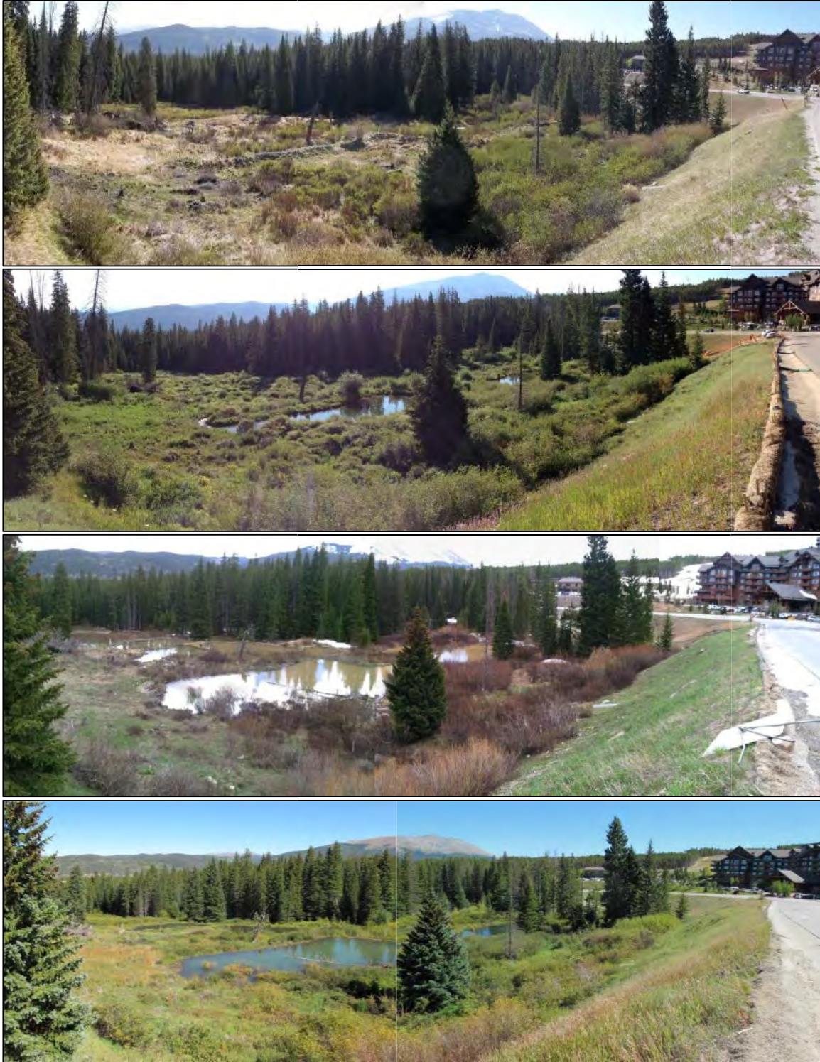
Figure 76: This series of photos shows a time lapse overview of a portion of the project area. Starting at the top, the photos are from (a) 2012 before the project, (b) 2013 after construction but before beavers arrived, (c) spring 2014 during runoff, and (d) summer 2014 after beavers significantly raised the height of dams.
