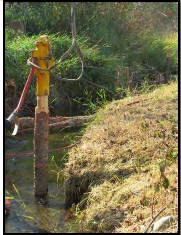
Figure 25: Hydraulic post pounder options. Options include, clockwise, starting from upper left: (a) a hand-held pounder attached to hydraulic power pack, (b) a post pounder attached to bulldozers, (c) a handheld pneumatic post pounder attached to an excavator and (d) a modified excavator with a vibrating pad. Options (a) and (b) take approximately 5 to 10 minutes per post, depending on substrate, and it can be difficult to get to the desired depth. Option (d) takes less than 1 minute per post and can drive posts as deep as needed. All pounders have a metal cylindrical cap that holds the post in place while pounding. Each option has pros and cons to consider, including cost, maximum depth the posts can be pounded, substrate type, operator strength and expertise, and the amount of likely riparian and instream disturbance. Photo credits: (a) Nick Weber, Ecological Research, (b) Mark Cookson, USFWS, (c) Peter Thamer, Siskiyou County Resource Conservation District, and (d) Julie Ashmore, Okanogan Highlands Alliance.
