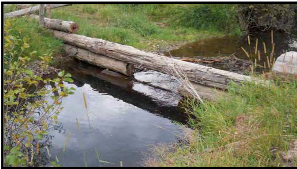
Figure 37: Flow-choke structures. These slow the movement of high-flow waters, increasing upstream flooding and creating temporary ponding, but during low flows they provide little functionality that is similar to a beaver dam. (From Devries et al. 2012).
