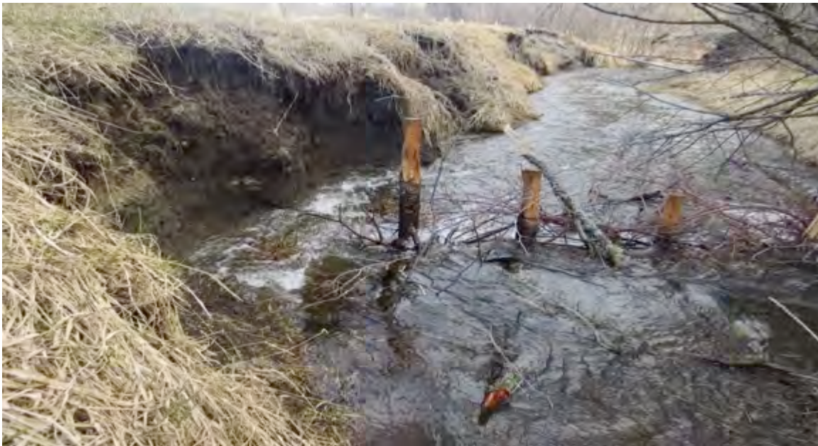
Figure 83: Breach of BDA 1 showing water flowing around the structure, eroding the left bank. This BDA is still functioning as grade control through water impoundment upstream as well as facilitating the widening of the incision trench. Notice the development of an inset flood plain directly downstream along the right bank
